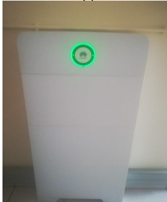
Figure 1.2 – 15kVA backup power inverter
